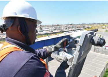
LED there be light in the 'Berg: The City's ongoing light-emitting diode (LED) streetlight installation and maintenance project is making steady progress. In Manenberg, with its approximately 200 streetlights along main roads, the City aims to replace older mercury-vapour installations with efficient, brighter LEDs over the coming months. Some R2 million has been budgeted for the refurbishment project, with the majority earmarked for Manenberg and Hanover Park. The aim is to increase area safety and complement crime prevention. Metro-wide, the programme will see more than 14 000 streetlights fixed this year.
