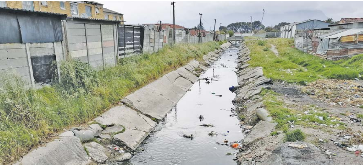
Can't go with this flow: One of the sections of the Manenberg canal that will be upgraded as part of the R50 million project to reduce pollution of the waterway and protect communities against flooding.
