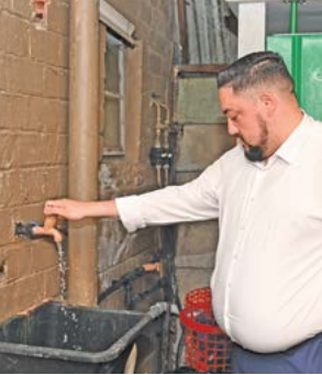
Tapped into services: Cllr Carl Pophaim (Mayoral Committee member for Human Settlements) inspects the services installed for several Hanover Park backyarders.
